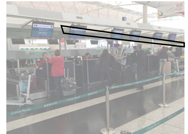
Drum louvers above at check-in islands
