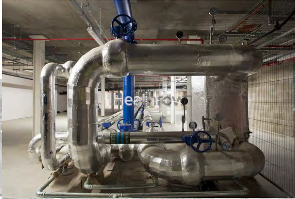
Duct supplying atmospheric air (denoted green on white)
