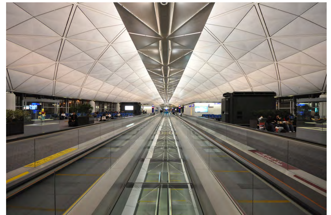
Glazing between the two moving walkways to allow light to enter the arrivals concourse
