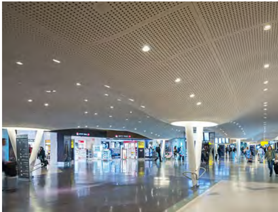
Combination of downlight recessed in undulating ceiling panels as well as hidden fixtures around structural columns
