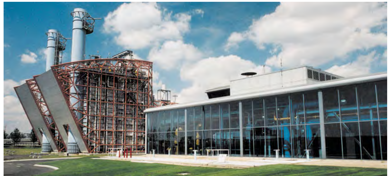
Kennedy International Airport Power Plant located in Jamaica, NY A gas-fired cogeneration facility that generates electricity and thermal energy for chilled and hot water
