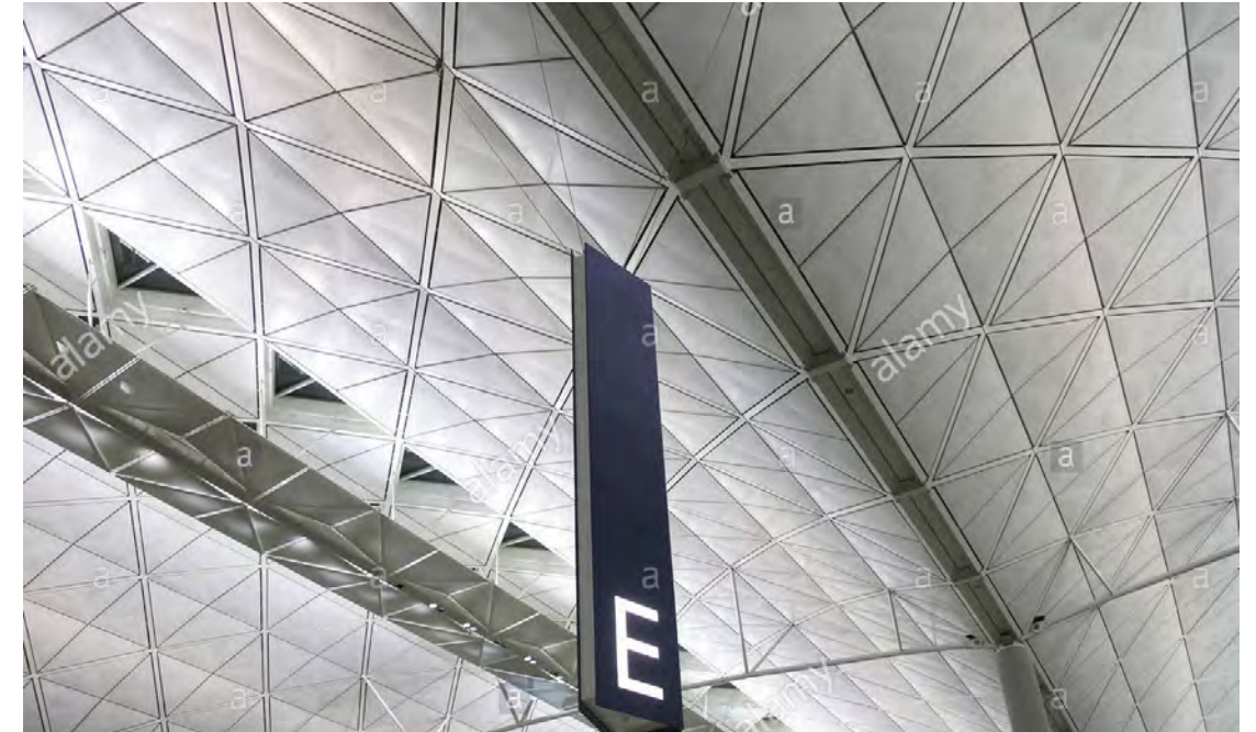
Effect of the lights reflecting off of the reflectors and roof at night
