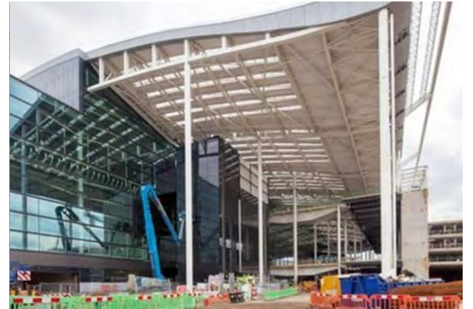
roof as shading device to allow for floor-to-ceiling east/west glazing
