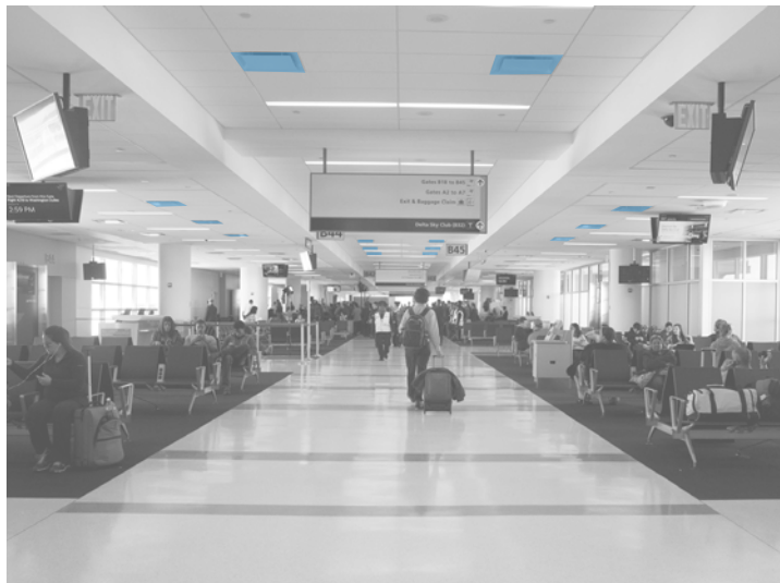
Drop ceiling grille along extension of concourse B
