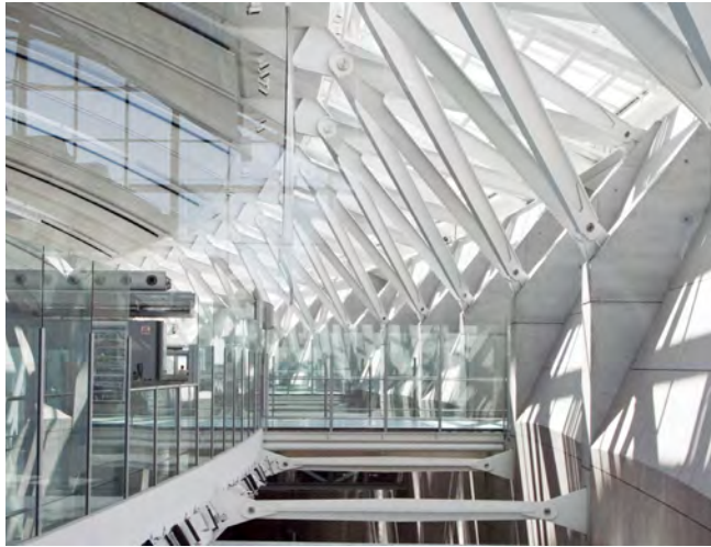
Daylighting for bridge from check-in to security (beneath is baggage claim)
