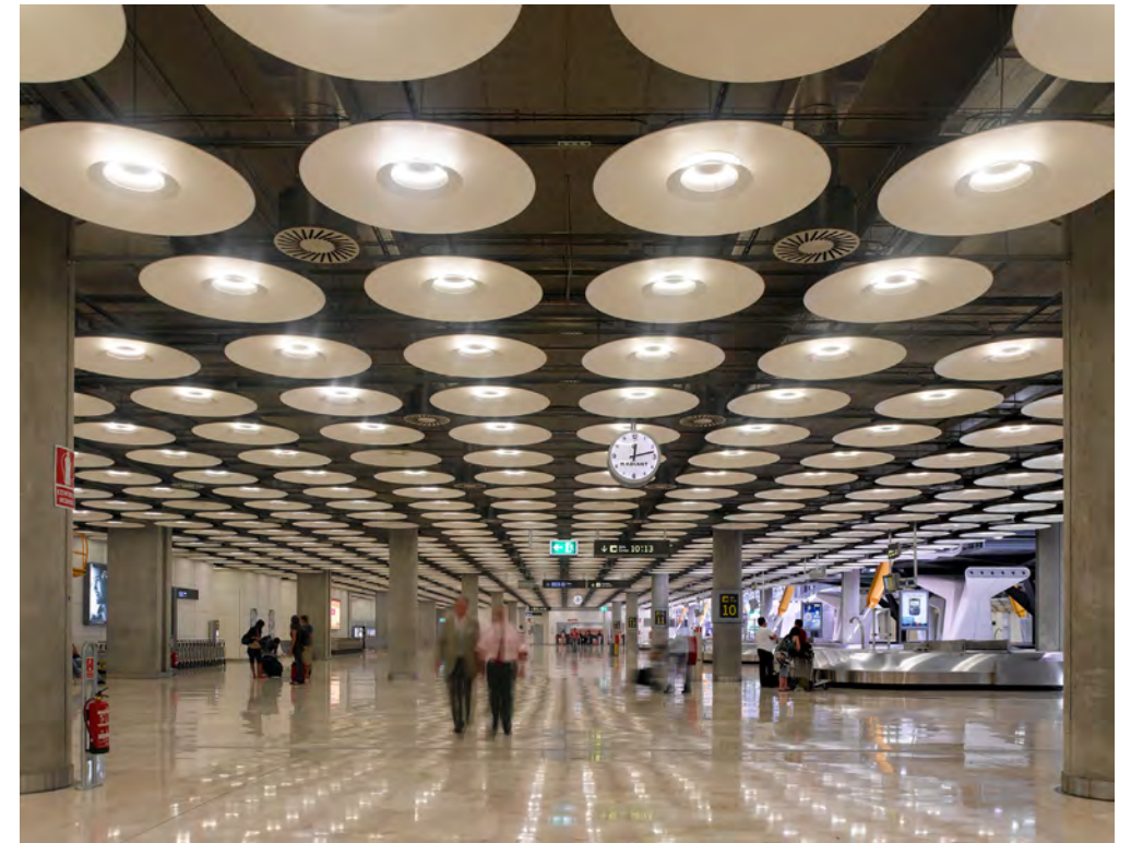
Lower level areas are illuminated by "the wok": provides downlighting, reflects light to distract from the concrete soffit/services and avoids need for suspended ceiling
