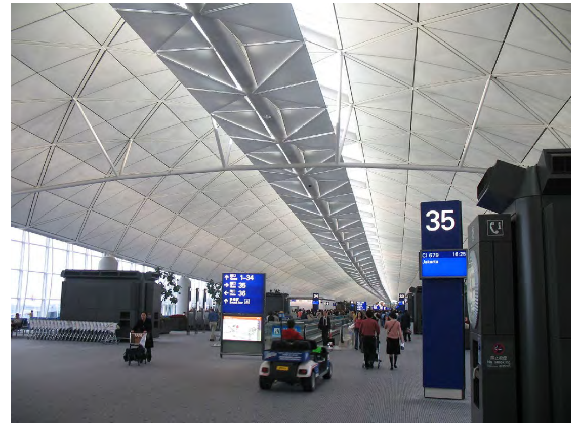
Reflectors along centre of roof to reflect diffused light into the space
