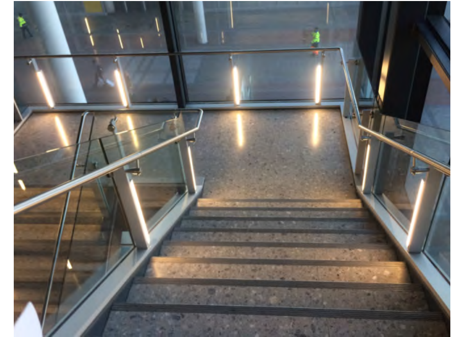
Vertical lighting along fire stair as a method for wayfinding
