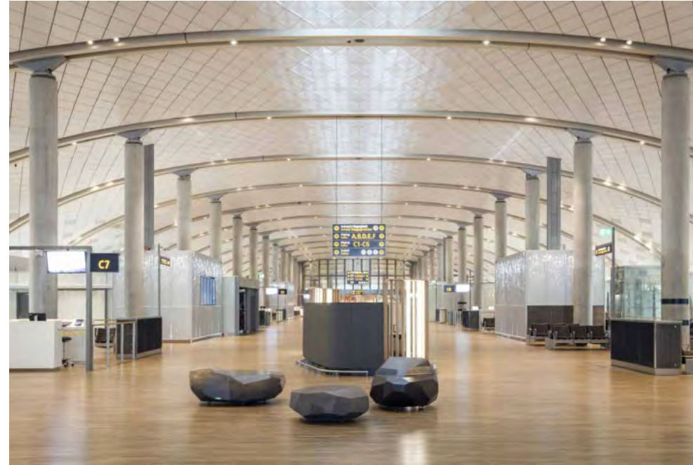
Skylights with translucent panels beneath to diffuse daylight
