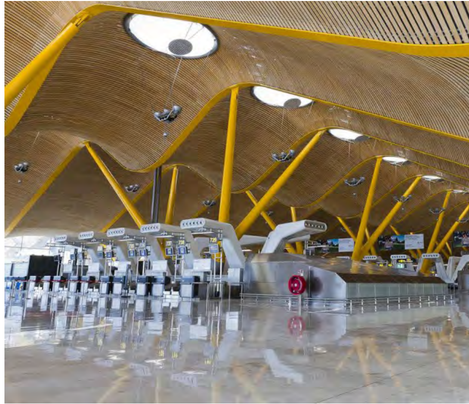
Daylight is diffused through the ETFE translucent layer
