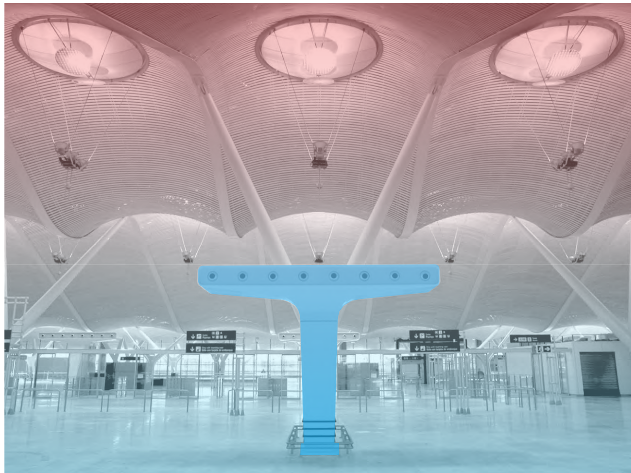
Displacement flow diffusers for high-velocity air ventilation & stratified (stacked) cooling system that extracts warm, stale air out near the ceiling
