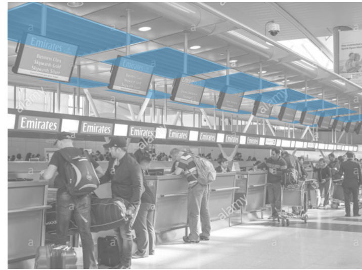
Drum louvers above check-in counters that ventilate (low speed, high volume)
