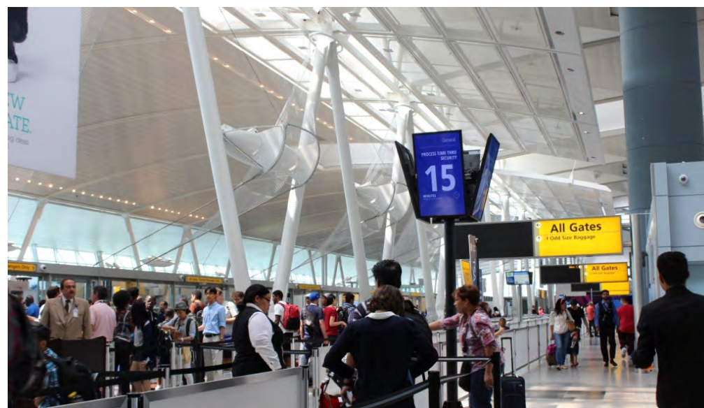
Perforated panels above security check-point that diffuses the light from clerestory
