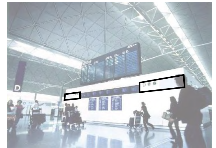
Jet nozzles at both ends of check-in islands
