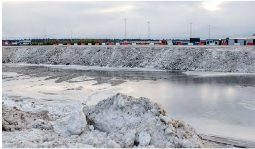
Snow Storage: snow will be covered with wood chip insulation once full
