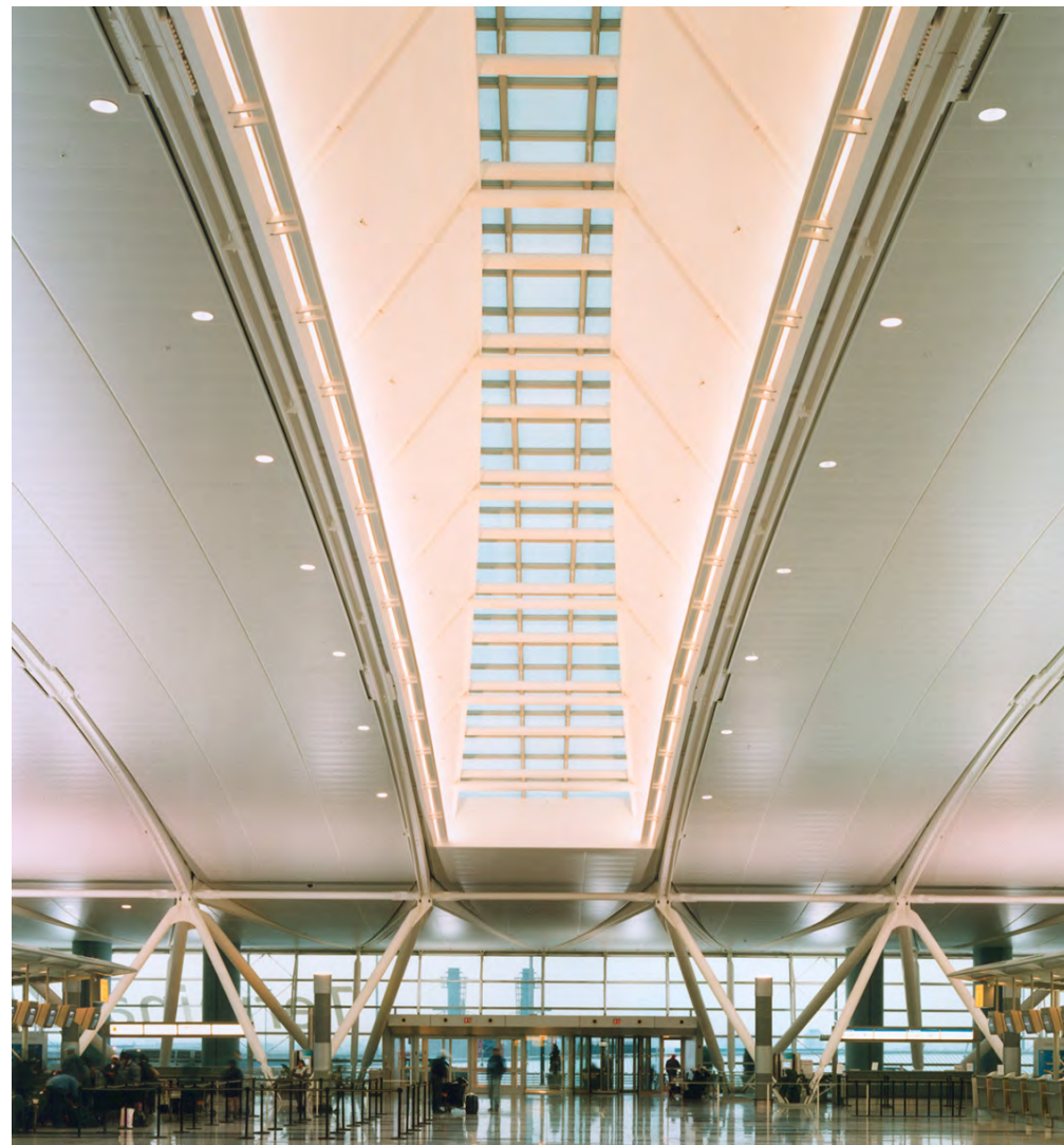
Skylights are wide and deep, allowing light to be diffused comfortably along the two sides before illuminating the space
